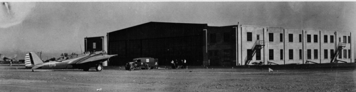
New hangar, new home: Servicing the first aircraft after moving to Denver Municipal Airport in early 1938. The new hangar was the nation's second largest NG aircraft facility.
